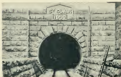
ST. CLAIR TUNNEL, SARNIA, ONT.
